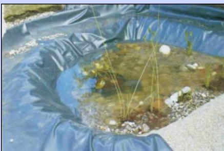
After gravel and plants are in place, at last it is time to put water in the pond: First fill it half full, then after the liner has settled completely, fill the pond.
