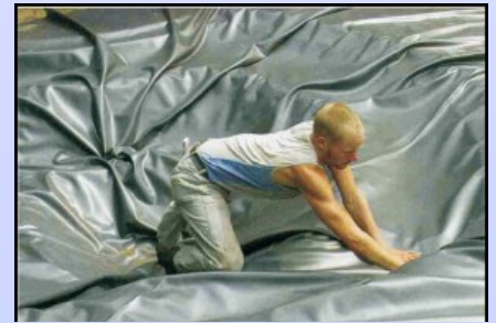
Then carefully lay out the liner.
